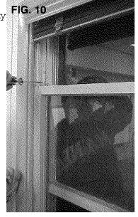
Out foam sash seal to window width and place into space between upper and lower sashes to seal out air infiltration
