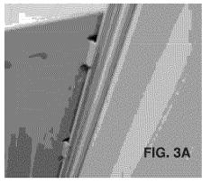
B. Slide the free end ("T"section) of the panel directly into the cabinet as shown in Figures 3A, 3B & 4. Slide the panel down. Be sure to leave enough space to slip the top and bottom of the frame into the rails on the cabinet.
