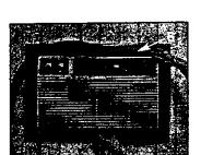
6. Install the 1"x 1½"x 84"long stuffer seal between the wall sleeve and the unit. A flat bladed screwdriver or putty knife is recommended.
