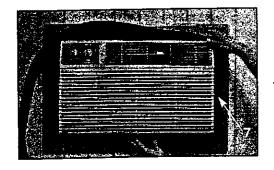
7. Install the 1"x 1½"x 84" long stuffer seal between the wall sleeve and the unit. A flat bladed screwdriver or putty knife is recommended.
