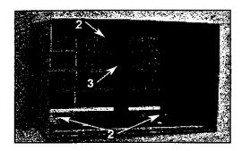
2. Attach the (2) 4½"x 3½"x 1½" foam blocks to the inside top and bottom of the wall sleeve with the slots 10" from the right side wall of the sleeve. Attach (2) Tapered Spacer Blocks behind rib on inside bottom of the wall sleeve as shown. Taper towards the rear of the sleeve.
