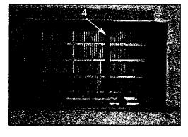
Install the new unit into the wall sleeve.Attach the ground wire to the unit as shown.
