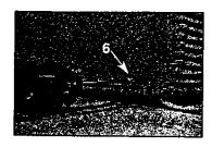
Install the new unit into the wall sleeve. Attach the ground wire to the unit as shown.
