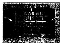
2. Cut (2) 17 Tapered Spacer Blocks to 13" and install as shown in the illustration with the tapered end ½ from the back of the sleeve.
