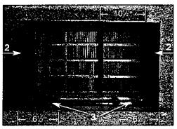
2. Attach the (2) 41/2" x 31/2" x 11/2" Centering/Support Blocks to the inside of the walls of the wall sleeve as illustrate with tapered end facing the opening of sleeve. These (2) blocks should be located approximately in the center of the side walls. To attach the blocks remove the backing paper from the blocks. Do not touch adhesive on the blocks. Press the blocks firmly in place.
