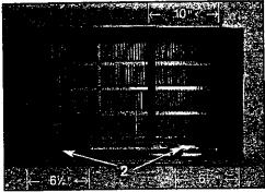
Attach (2) Tapered Spacer Blocks to the inside of the wall sleeve as shown in the illustration. DO NOT CUT THESE BLOCKS.
