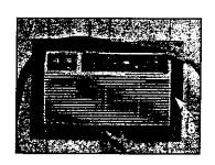
8. Install the 1"x 11/2"x 84" long stuffer seal between the wall sleeve and the unit. A flat bladed screwdriver or putty knife is recommended.
